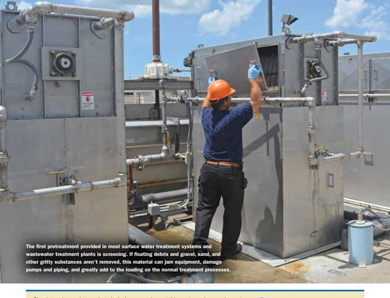
Clogging and corrosion are the principal problems associated with screening. Preventing these problems requires routine cleaning and inspection. Consider the following guidelines:
