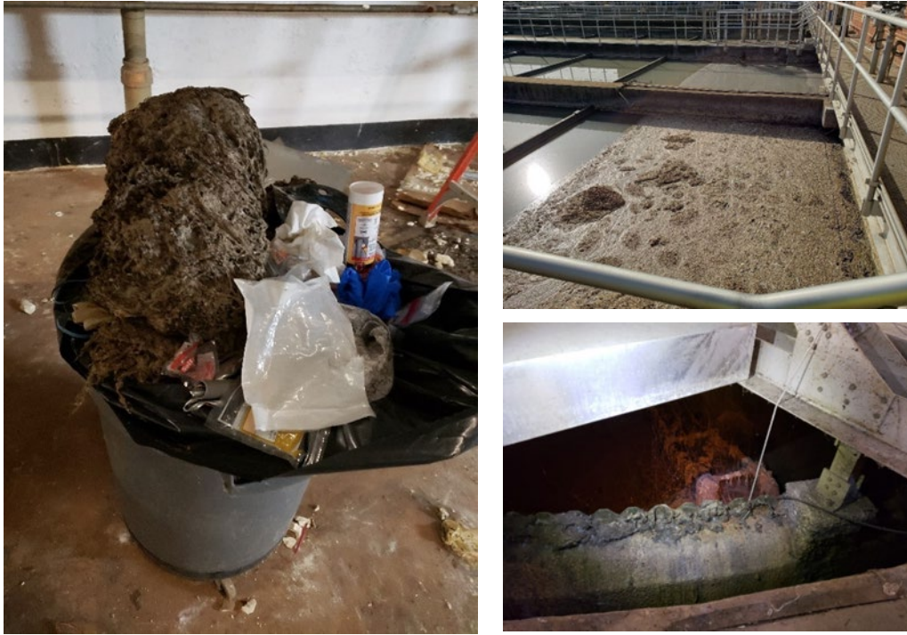
Figure 1 Materials Passing Downstream of the Screens
